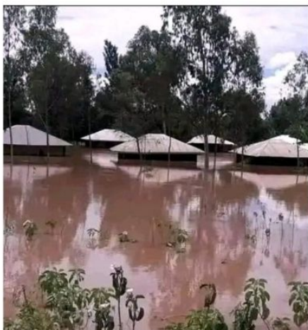
Houses in some parts of Kisumu where floods were rampant
