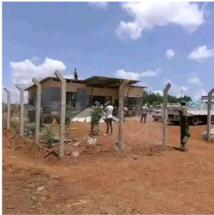
House construction ongoing in Kelvin Kiptum's home | Photo Courtesy
